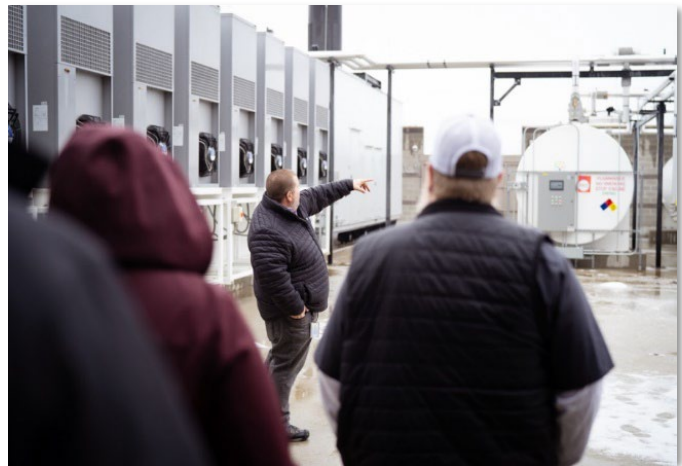
Tour of Sabey Data Centers in East Wenatchee, Douglas County
