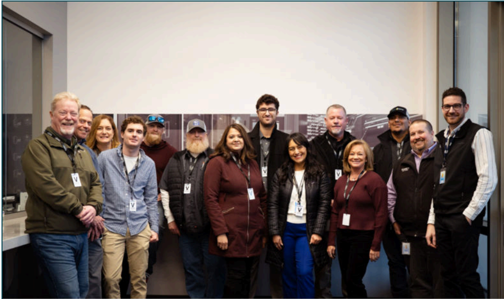
SkillSource Board Member and VP of Sabey Data Centers West, Ryan Beebout, gives a tour of Sabey Data Center in East Wenatchee.
